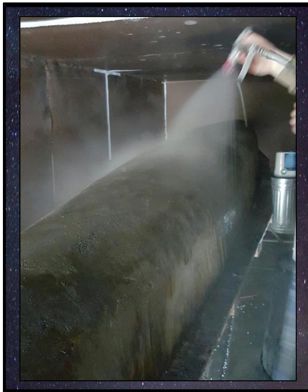
Figure 20: Applying Sealer
