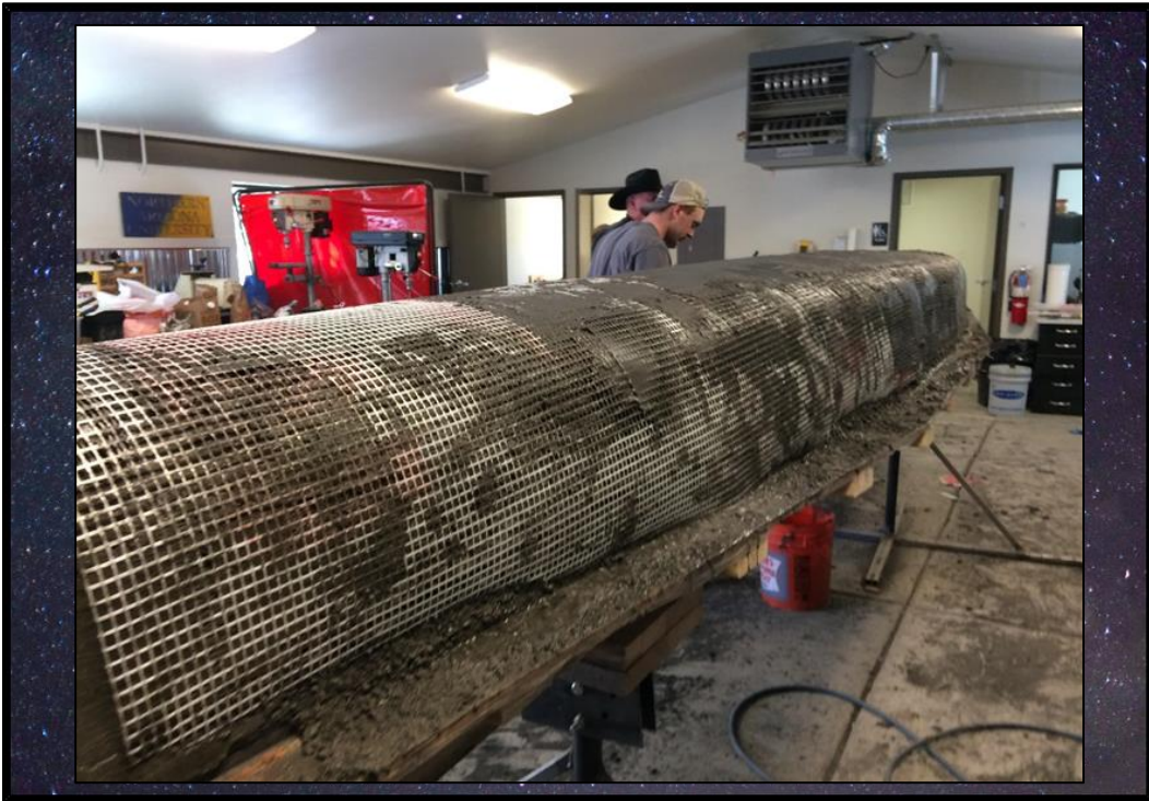
Figure 14: Placing Reinforcing Mesh over Canoe
