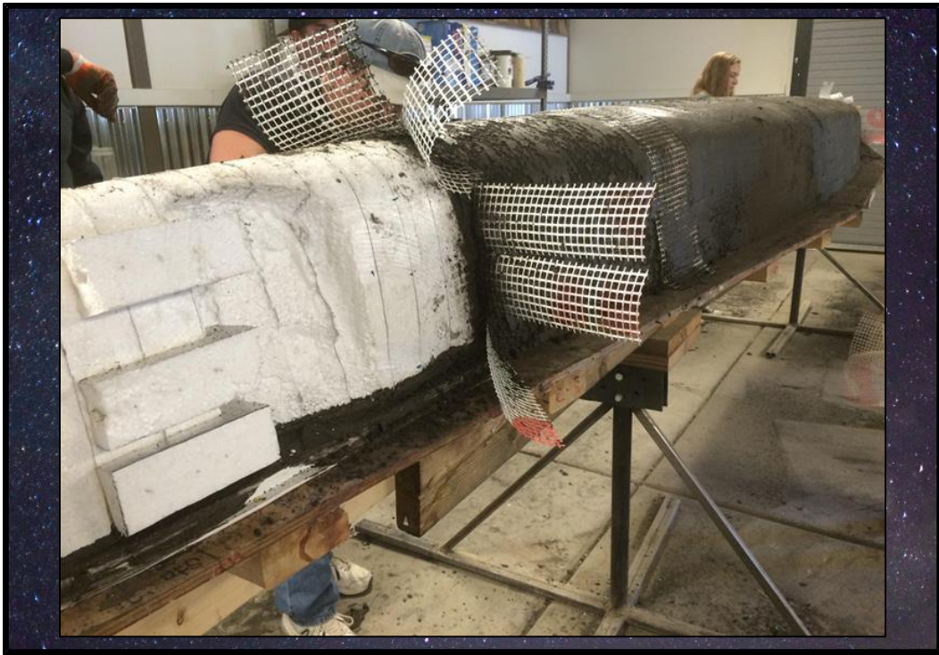
Figure 13: Placing Reinforcement on Stern Bulkhead
