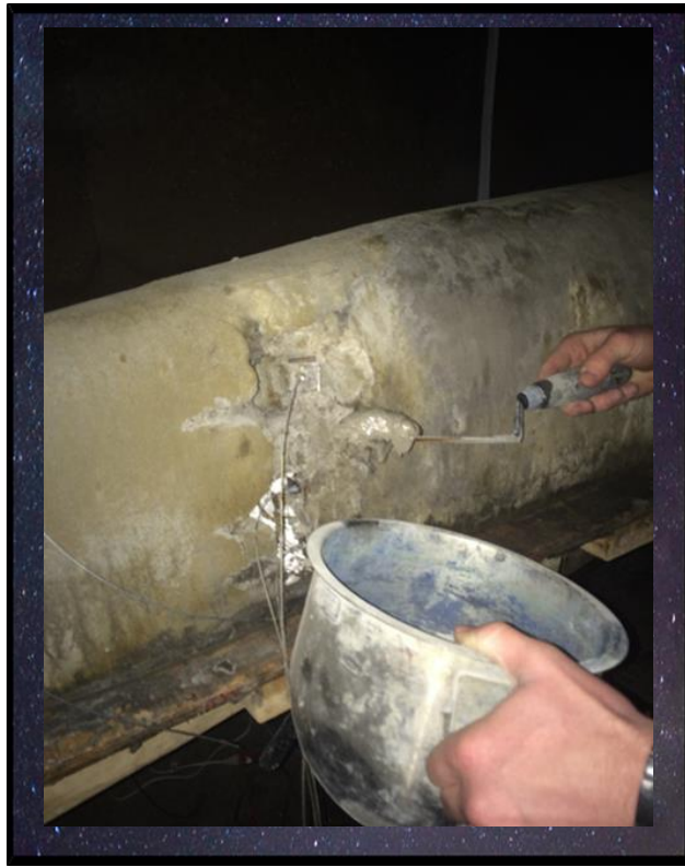
Figure 17: Placing Concrete in Post-Tensioning Void
