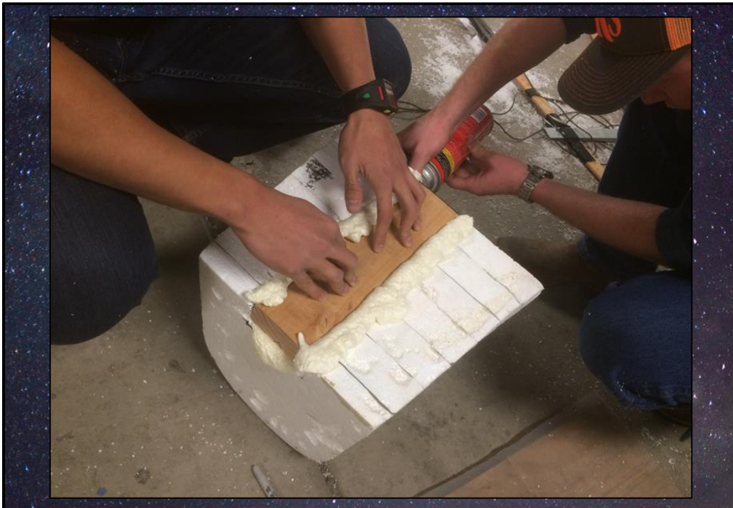
Figure 4: Placing Wood in Cross-Section
